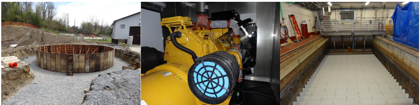
Above: Interior picture of our new
