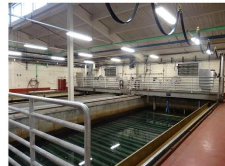
Two refurbished Filters (Filters #1 & #2)
